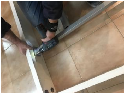
ASSEMBLY METALLIC CROSSBARS WITH SIDERAILS
